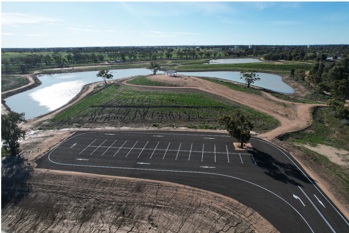
Figure 2: The new wetlands carpark is complete
