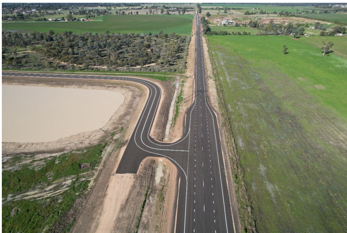
Figure 8: Sealing and linemarking of Gainsborough Road is complete
