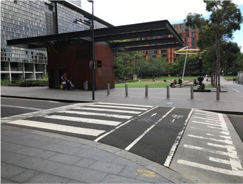
Figure 4.6 Pedestrian crossing with bicycle space allocated beside it, Chippendale Way, Chippendale Pedestrian ramps
