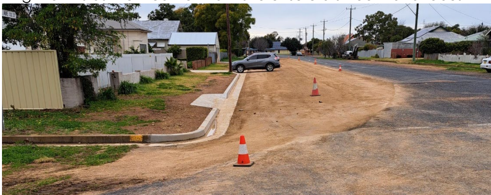
Figure 4: Kerb and gutter has been installed along Fourth Ave
