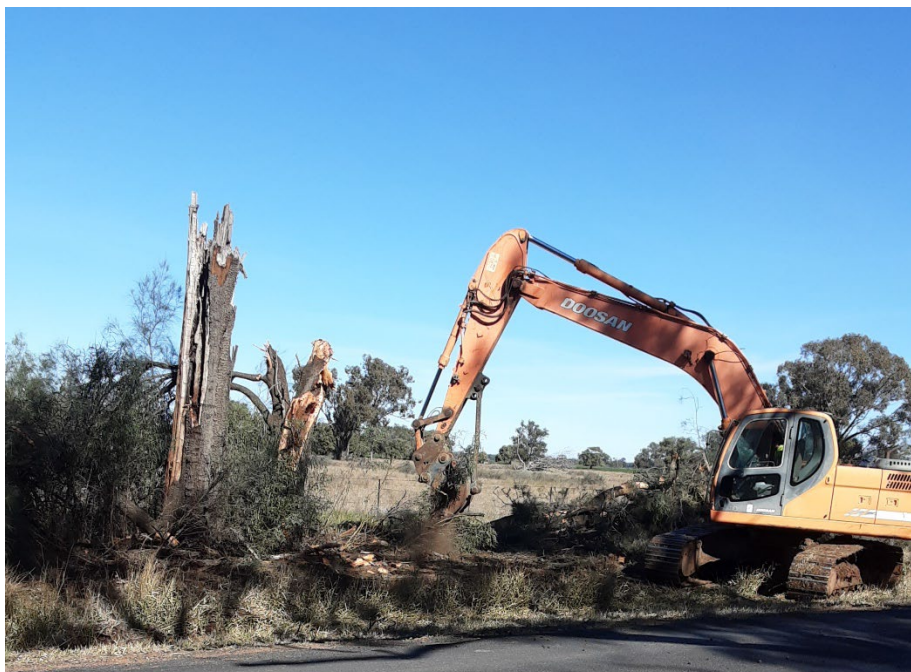
Figure 5: Tree Removal on Enmore Road
