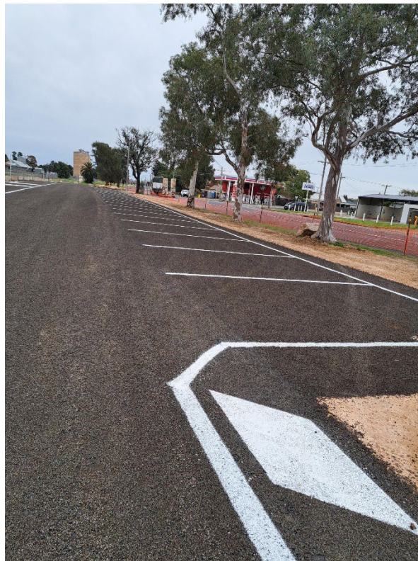
Figure 7: Burraway Street Carpark has been sealed and line marked
