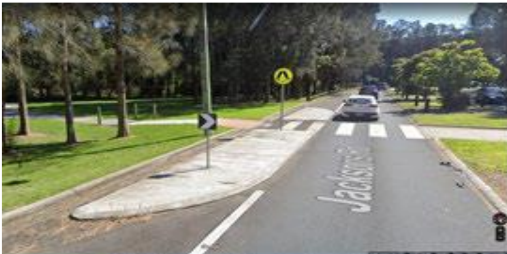
Figure 4.5 Kerb blisters, Jacksons Road, North Narrabeen
