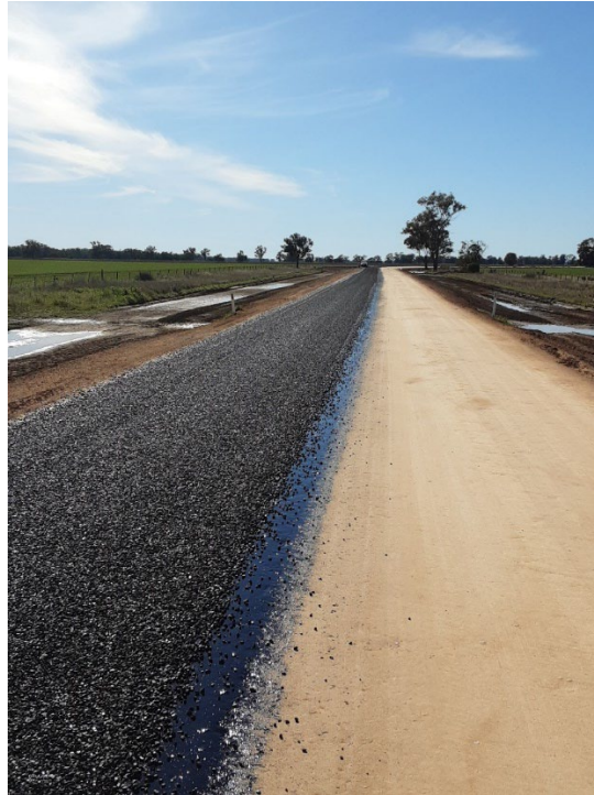
Figure 6: Enmore Road has recently been sealed
